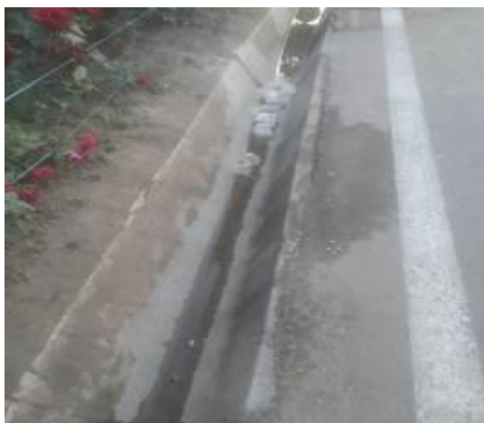
Figure 2: disposal of polyethylene waste into the drainage system
